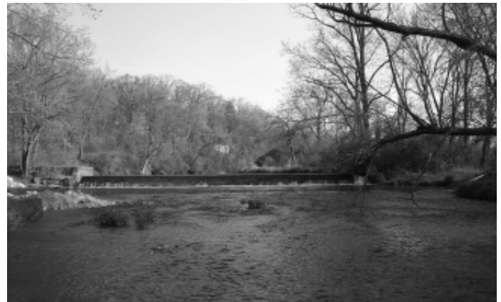
The newly built fish passage over the Big Rock Creek Dam in northeastern Illinois. (Photo courtesy of Steve Pescitelli)
